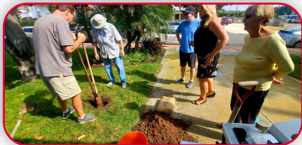
Breaking Ground for Our Little Library
